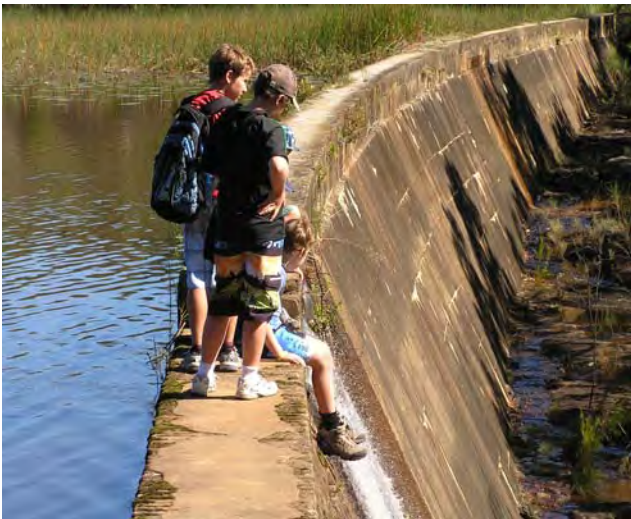
Dam wall forming Lake Toolooma
